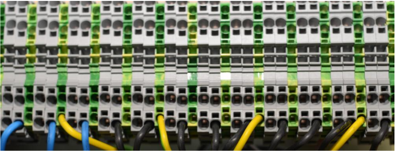
Figure 2.3.13. The upper panel with the RPCM DELTA terminals (fragment).
