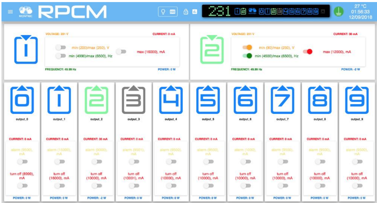
Figure 4.2.17. The Dashboard control panel in the Show Limits mode RPCM with ATS.
